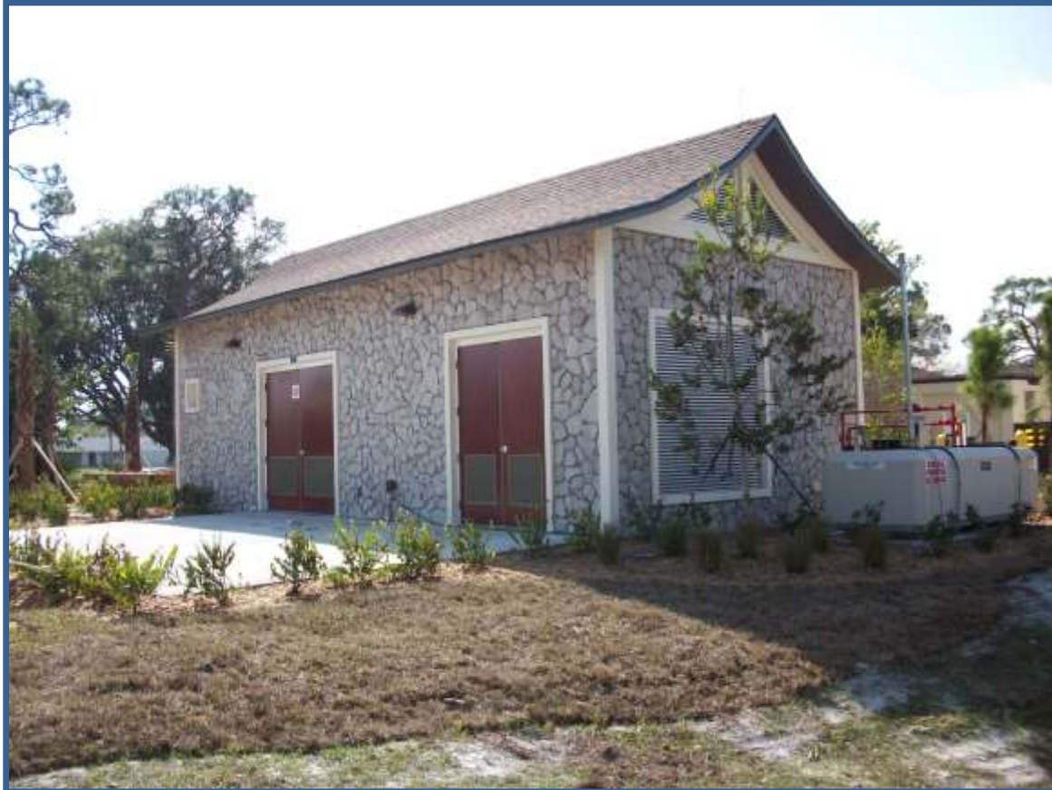
North River Shores Wastewater Vacuum Building
