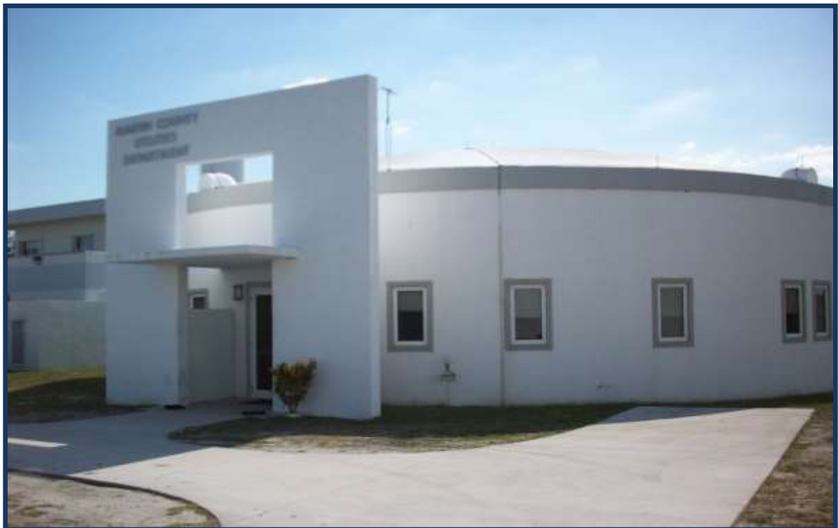
Field Maintenance Building (Converted Water Tank)
