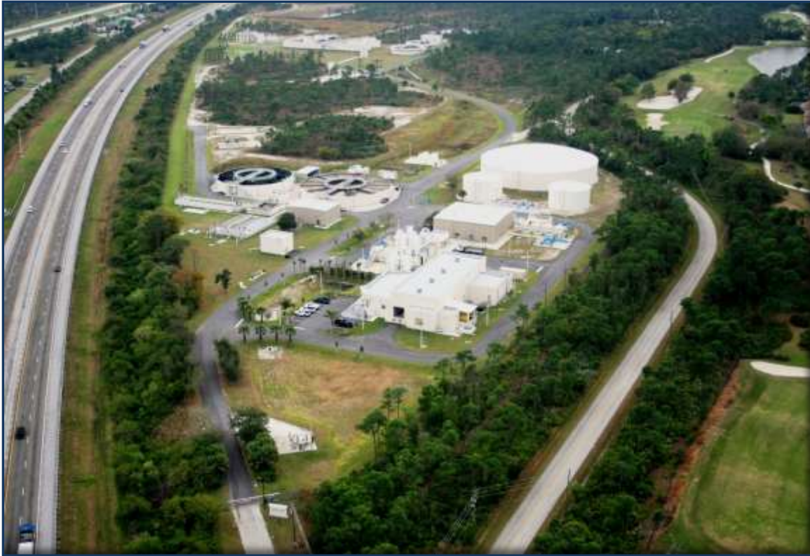
Tropical Farms Treatment Facility
